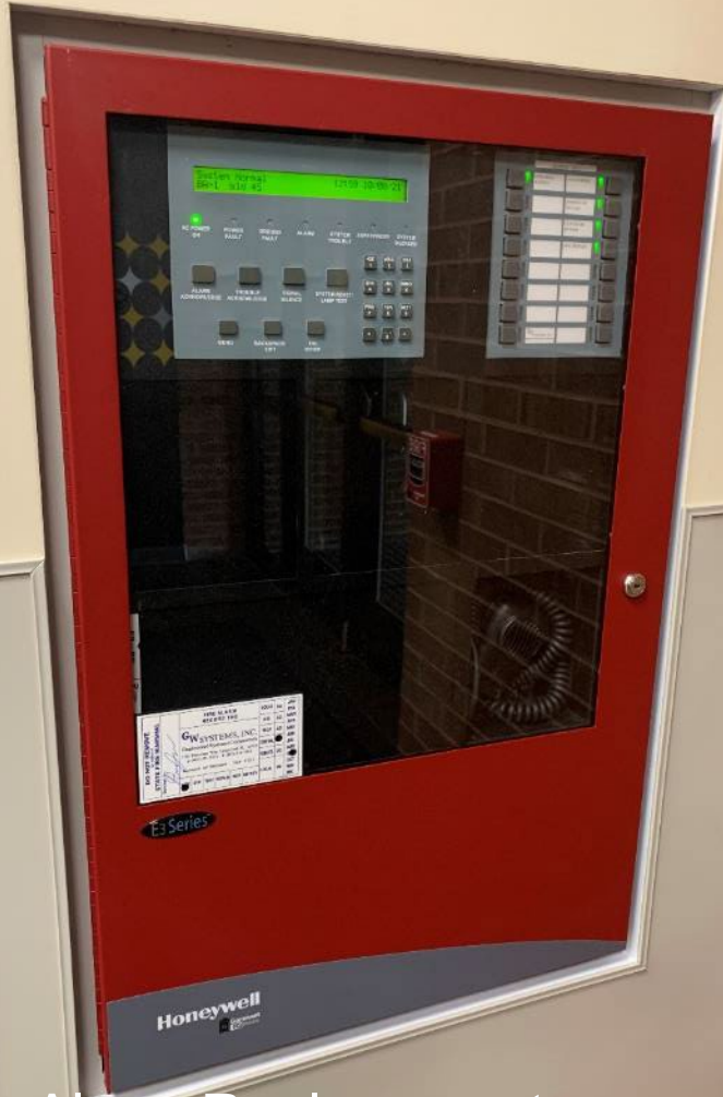
Fire Alarm Replacements
